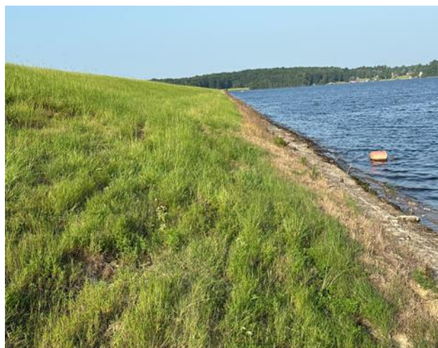
Upstream Embankment Photo
