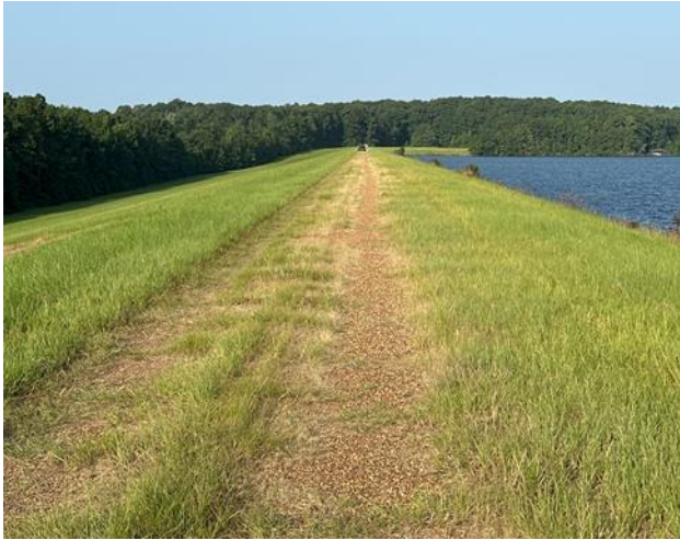
Embankment Crown Photo
