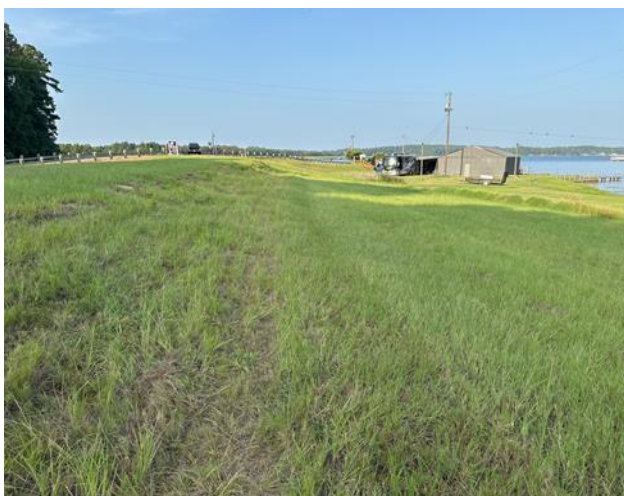
Upstream Embankment Photo
