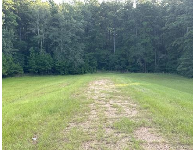
Embankment Crown Photo
