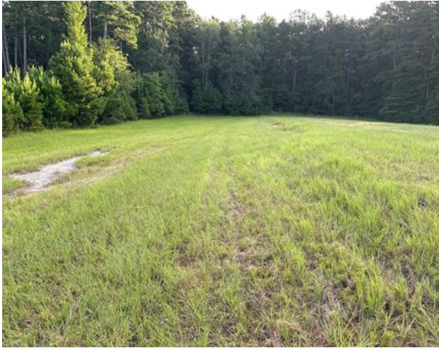
Upstream Embankment Photo
