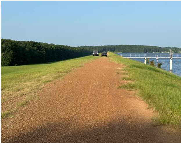
Embankment Crown Photo
