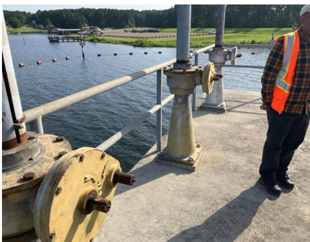
Outlet Works Photo
