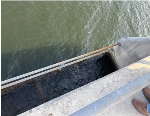
Outlet Works Photo
