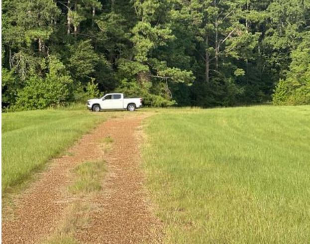
Embankment Crown Photo
