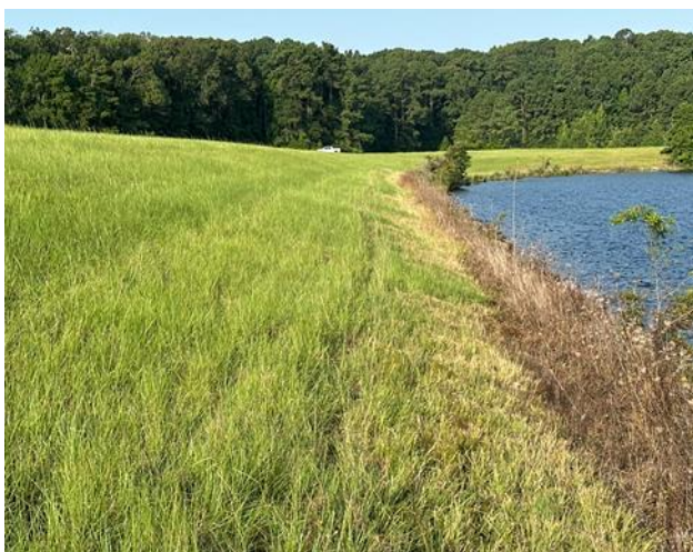
Upstream Embankment Photo
