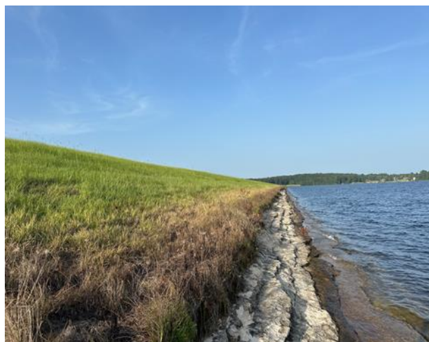
Upstream Embankment Photo
