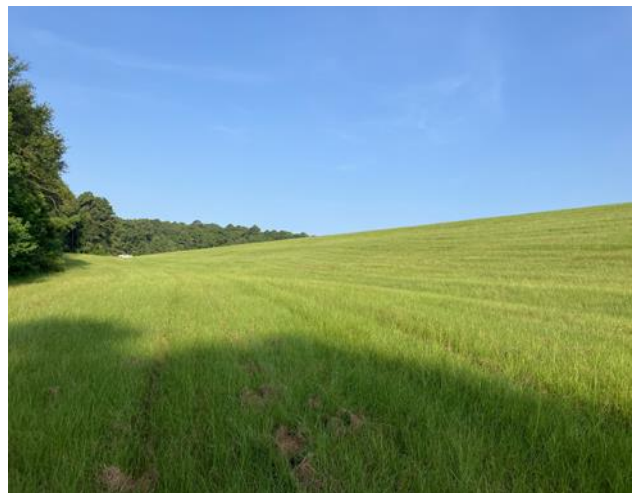
Downstream Embankment Photo
