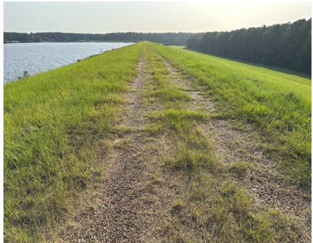
Embankment Crown Photo
