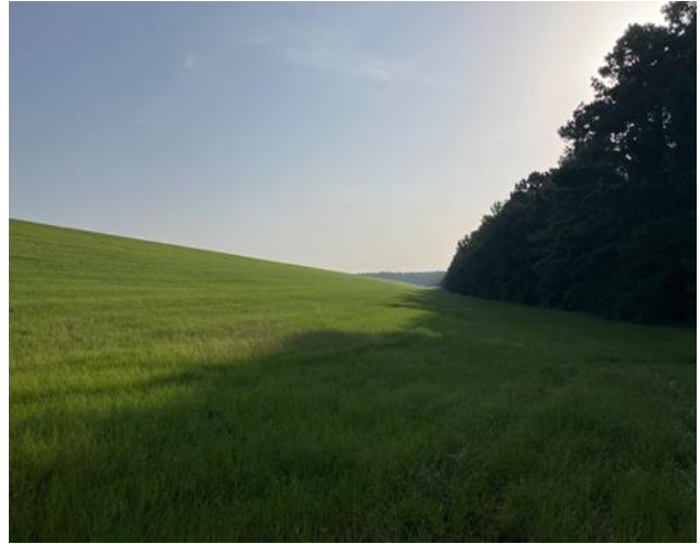
Downstream Embankment Photo
