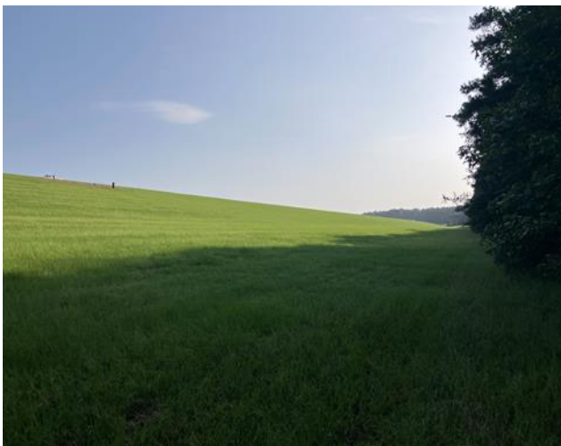
Downstream Embankment Photo
