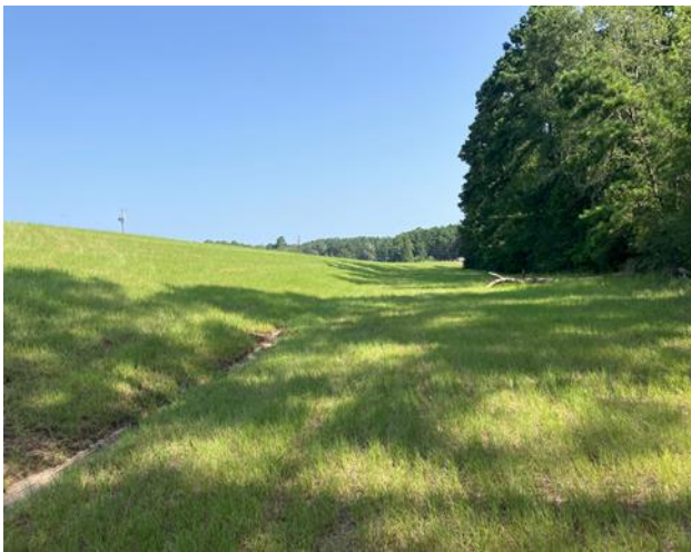
Downstream Embankment Photo
