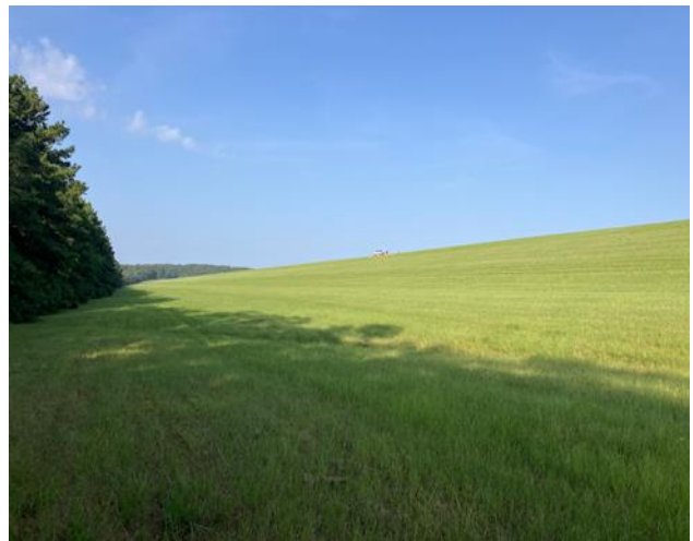
Downstream Embankment Photo
