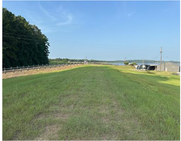
Embankment Crown Photo
