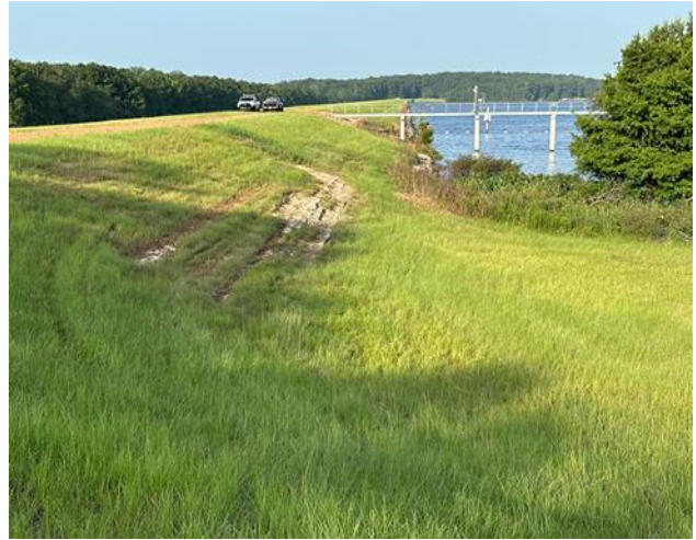
Upstream Embankment Photo
