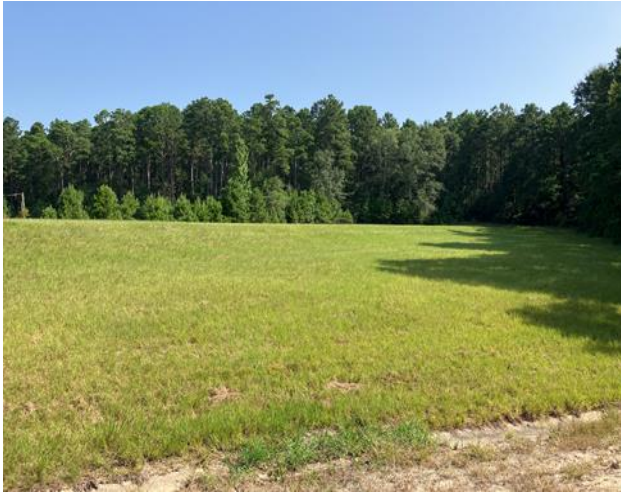
Downstream Embankment Photo
