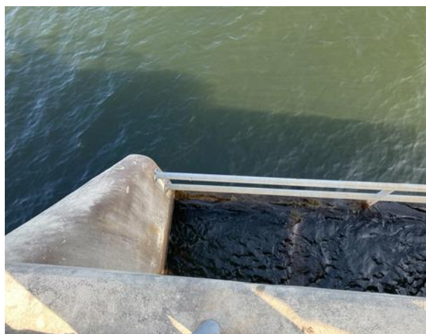
Outlet Works Photo
